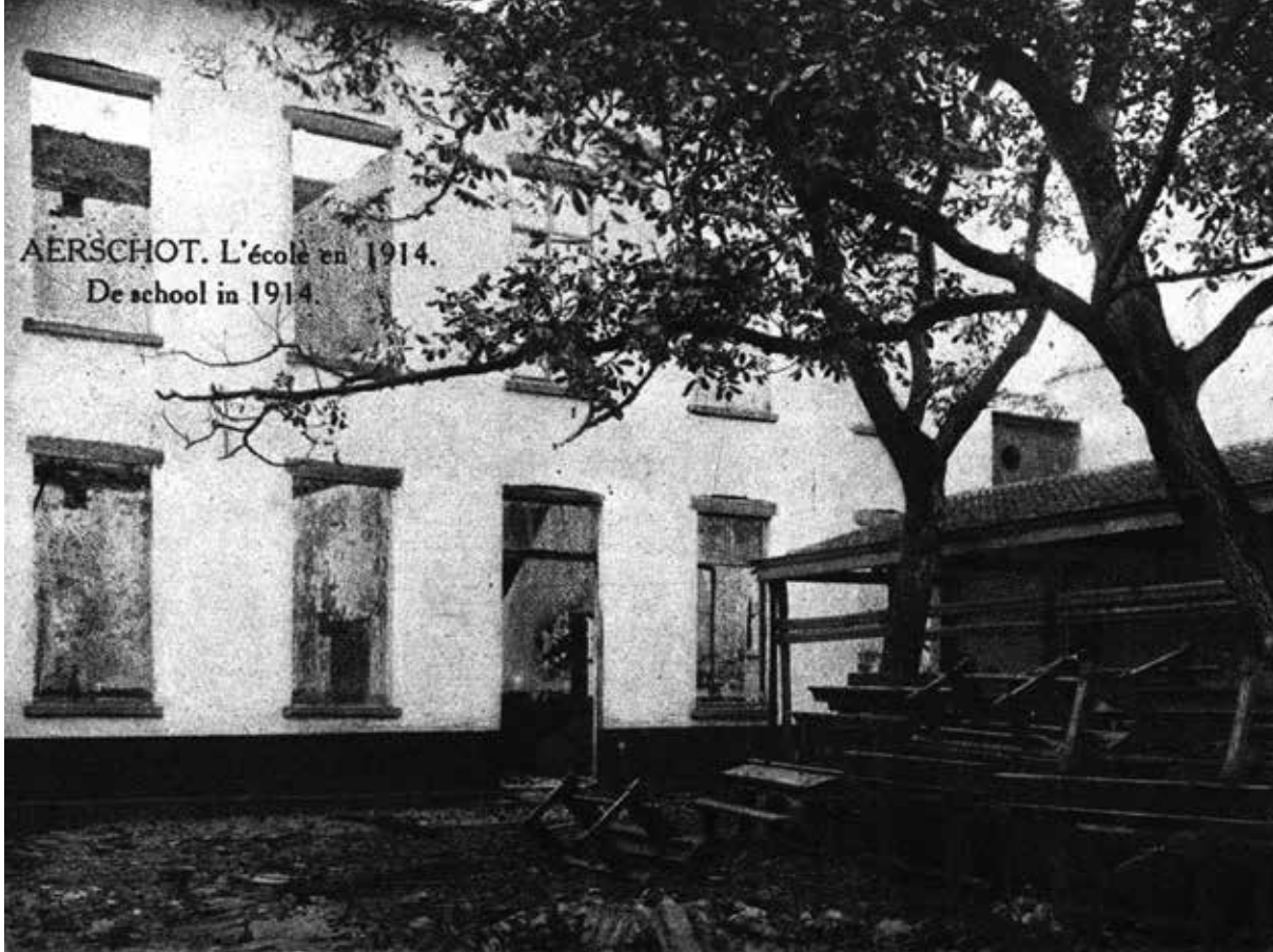
Verwoeste school in Aerschot.
